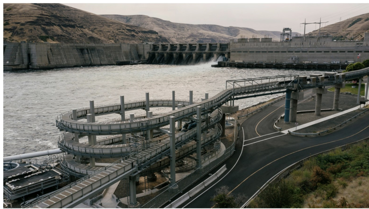
A juvenile salmon capture and transport structure at Lower Granite Dam, one of the four Lower Snake River dams. Despite such efforts, multiple salmon runs on the river are veering toward extinction.
