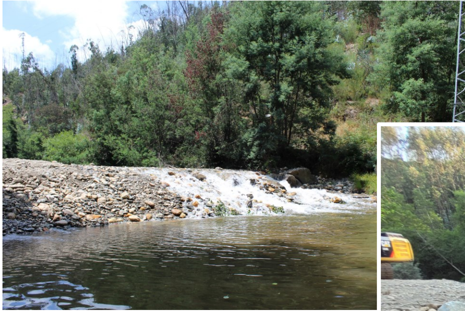
Redonda weir (downstream) River Águeda
