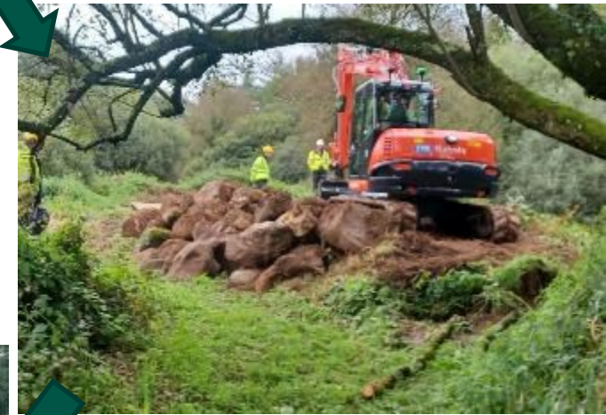
Previously dredged boulders going back in
