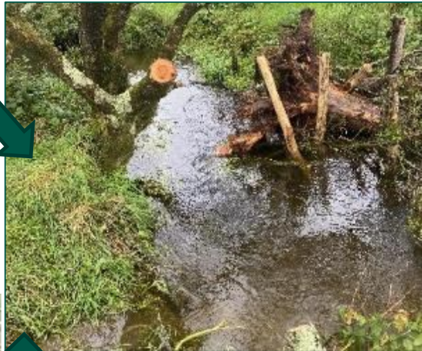
Adding wood to a straightened channel
