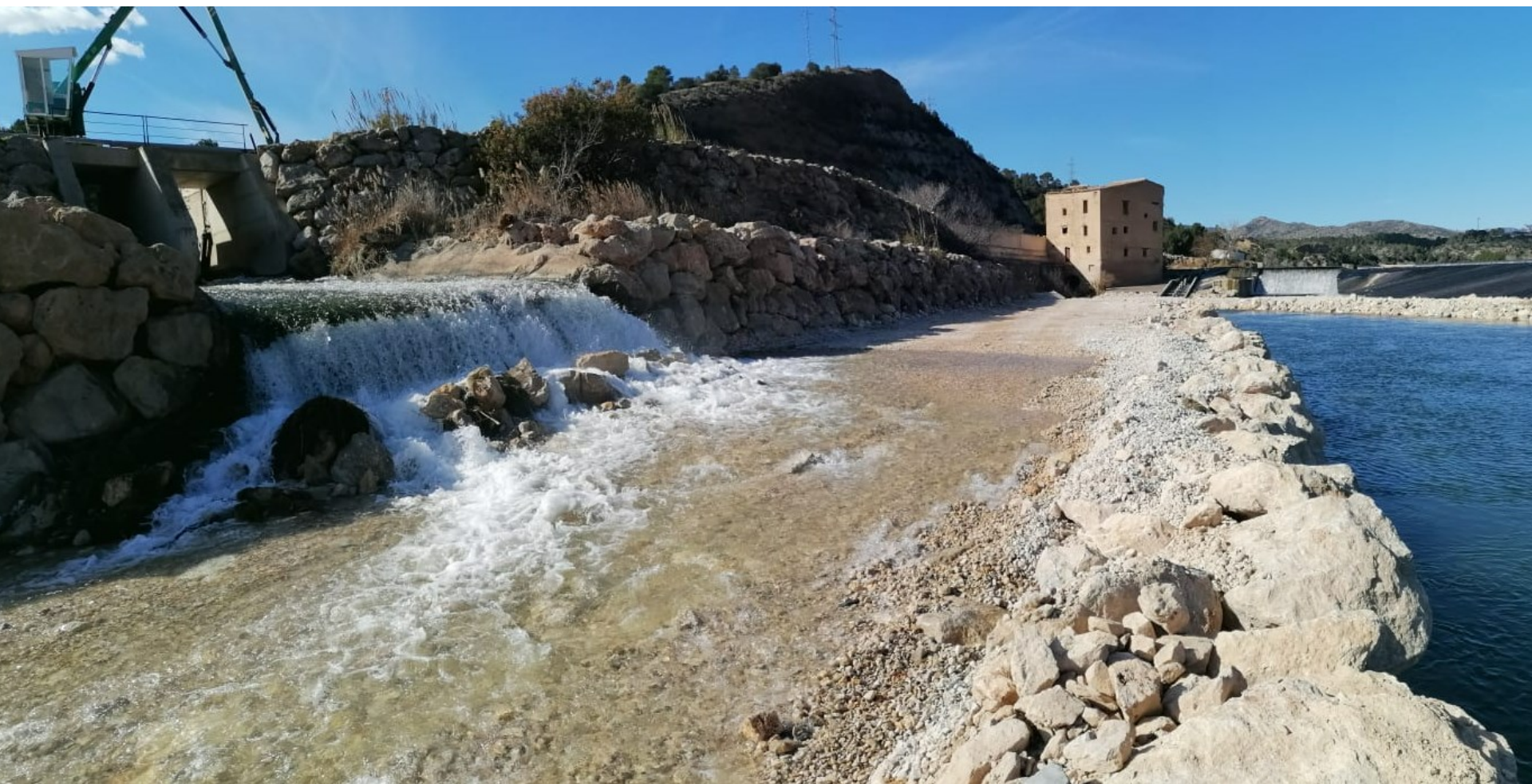
Xerta fish ramp. Building in process (picture of Marc Ordeix from 2024/02/13)
