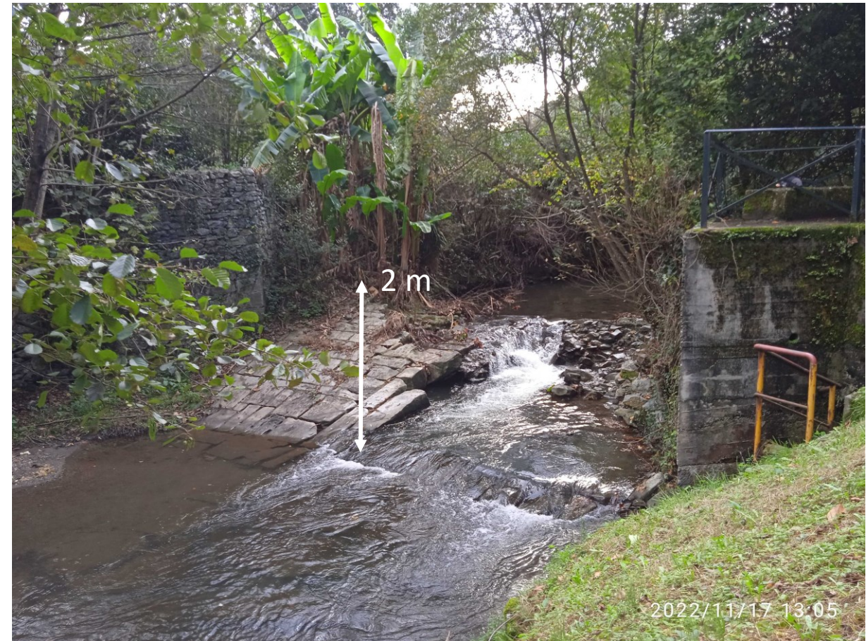
Beheko Errota Mill dam (Onin)
