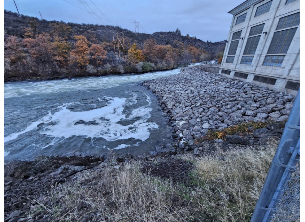
Copco 2 tailrace backfilled with rip rap 11 November 2023
