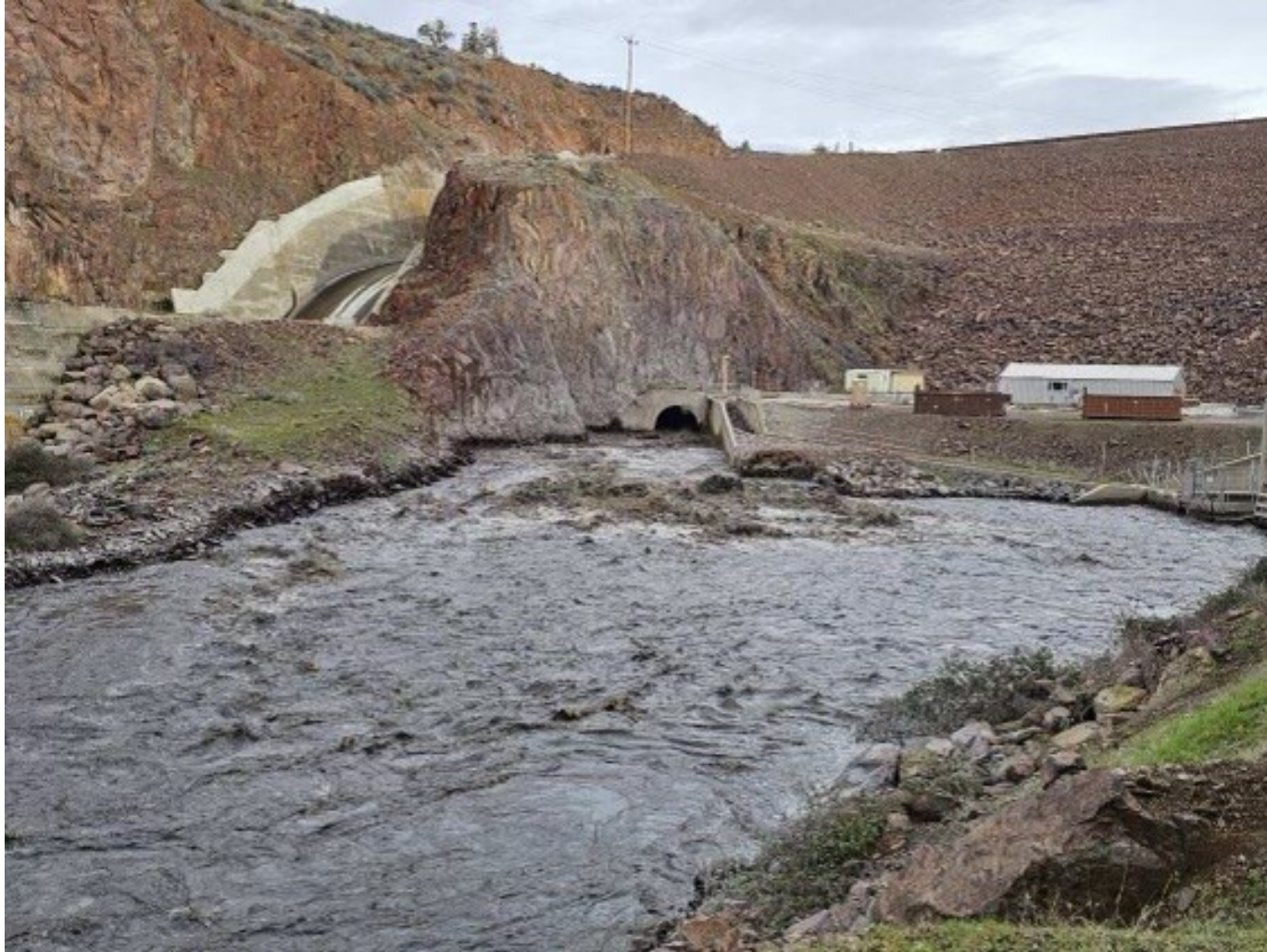
Klamath River at Low Level Outlet tunnel. 5 February 2024
