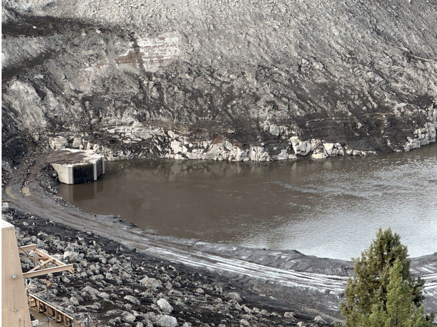
Exposed diversion tunnel intake structure trash racks at Iron Gate. 12 March 2024
