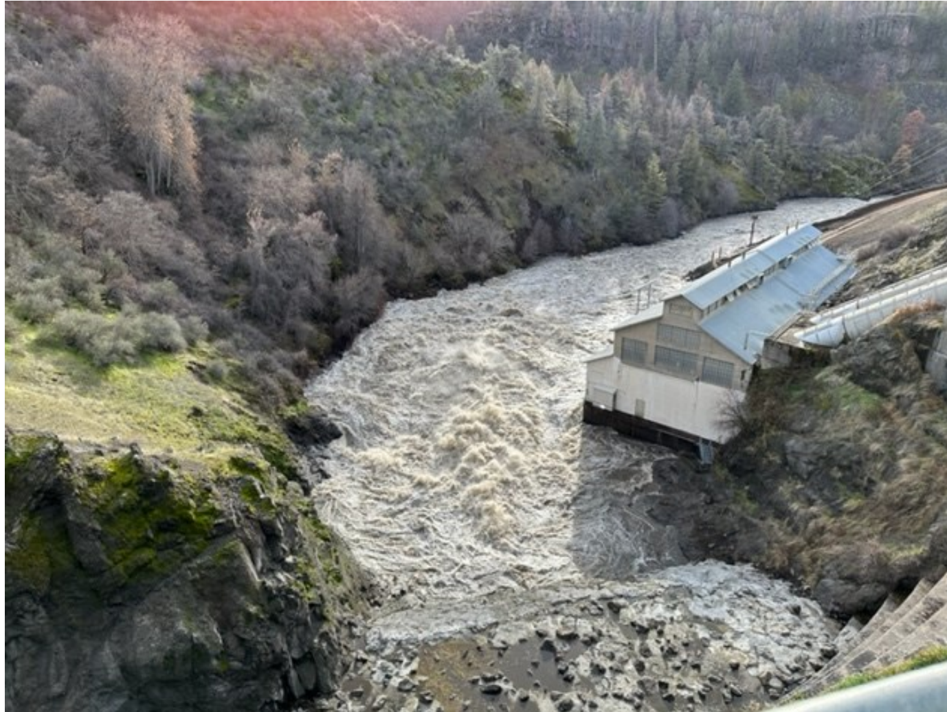
View of Copco No. 1 Powerhouse and river channel after adit plug blasted 23 January 2024
