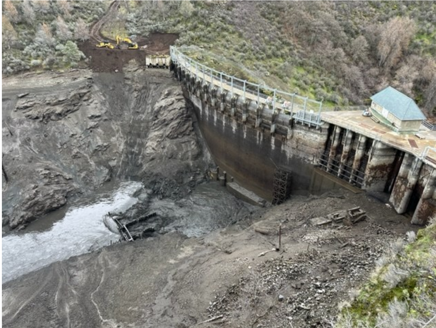
View of Copco No. 1 Dam and reservoir after drawdown. 31 January 2024
